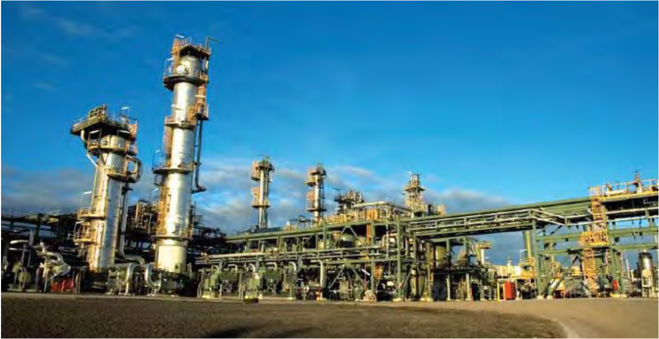
Processing plants, called trains, at Gladstone and Curtis Island will convert coal seam gas to LNG *
