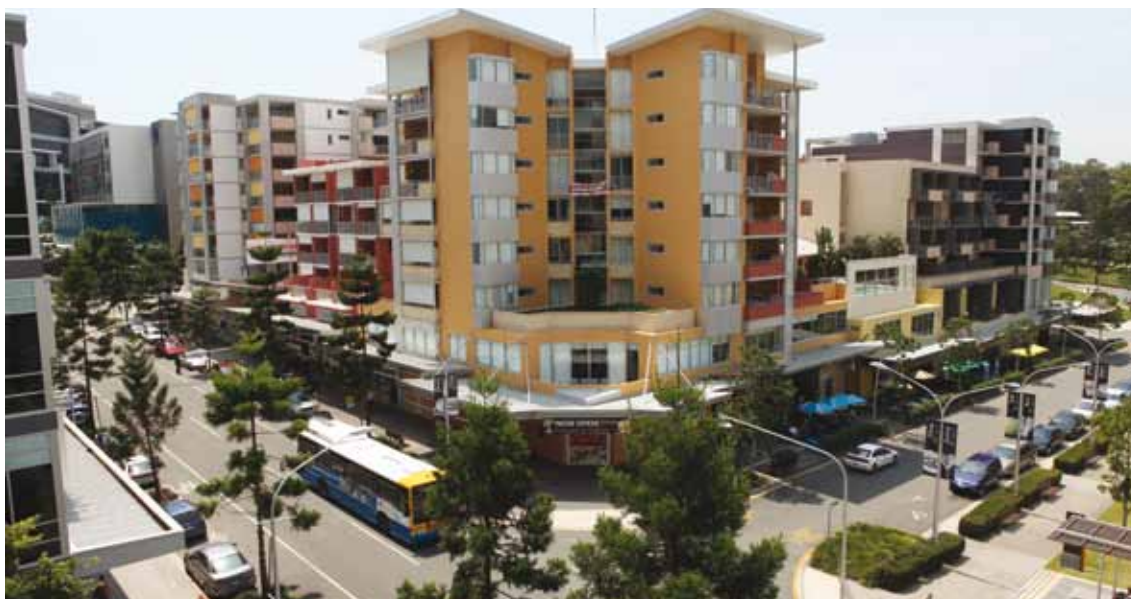
Kelvin Grove Urban Village, Brisbane – demonstrates the application of a number of transit oriented development principles. The village comprises a mix of uses, provides a high-quality public domain and access to public transport.
