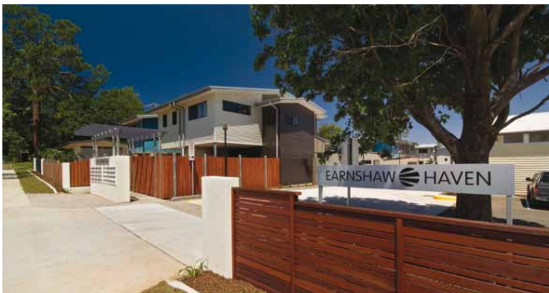
Earnshaw Haven, Nudgee, Brisbane (Brisbane Housing Company) – provides a variety of tenure options, including affordable rental housing as well as market housing (developed as a master-planned community).
